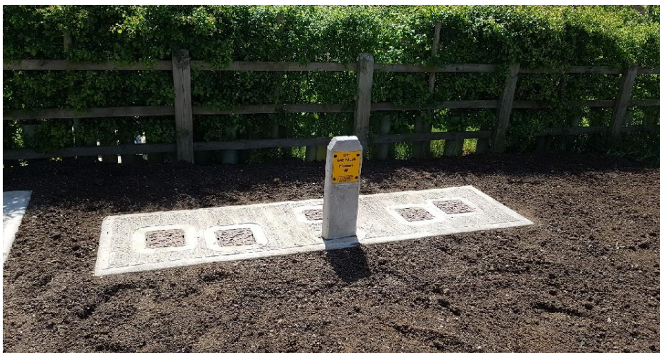
Figure 40 – An example of how the valve nest should be finished
