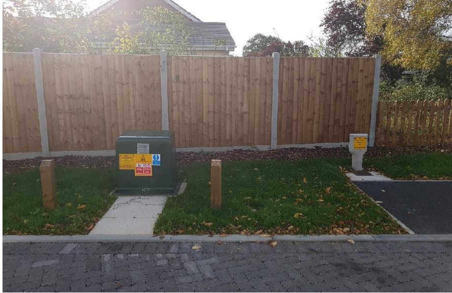
Figure 39 – An example of how a small above ground installation should be finished
